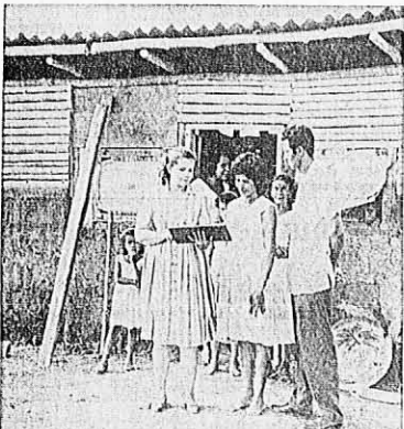
IMPROVED HOME—Leaders of the community development project outside David, Panama, talk with Elvia, center, about her third home. The building in the background is the improved home built on property she got under a government land reform program. A concrete block home (two bedrooms) value $500 will be built in front of this present structure.
