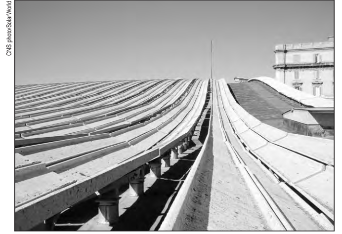
This photo montage provided by SolarWorld shows how solar panels will look on the roof of the Vatican's audience hall when installed in 2008. Some 2,000 panels were donated to the Vatican by SolarWorld, a German company.
