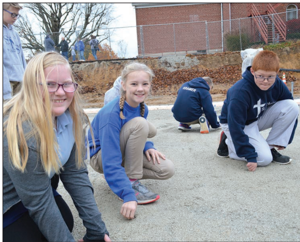
Mary Schmidl, left, Lilah Butz and Henry Schneider, all sixth-graders at St. Nicholas School in Ripley County, place blessed medals of saints in gravel on Nov. 5, 2018, where a foundation was later laid for a new education center at the Batesville Deanery faith community. (Submitted photo)
